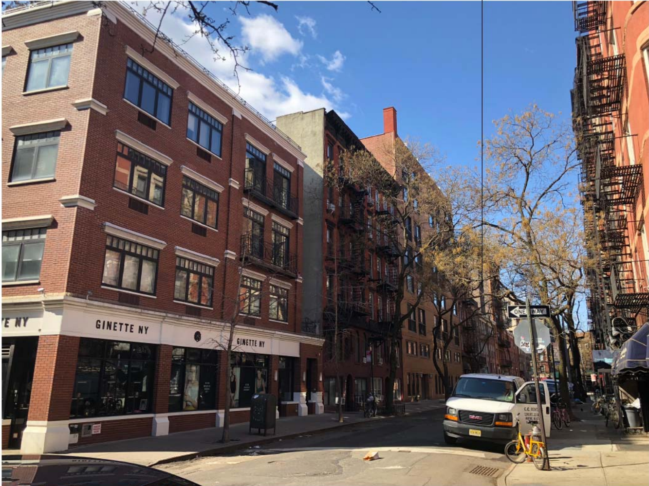
3. View from NE corner of Bleeker street
