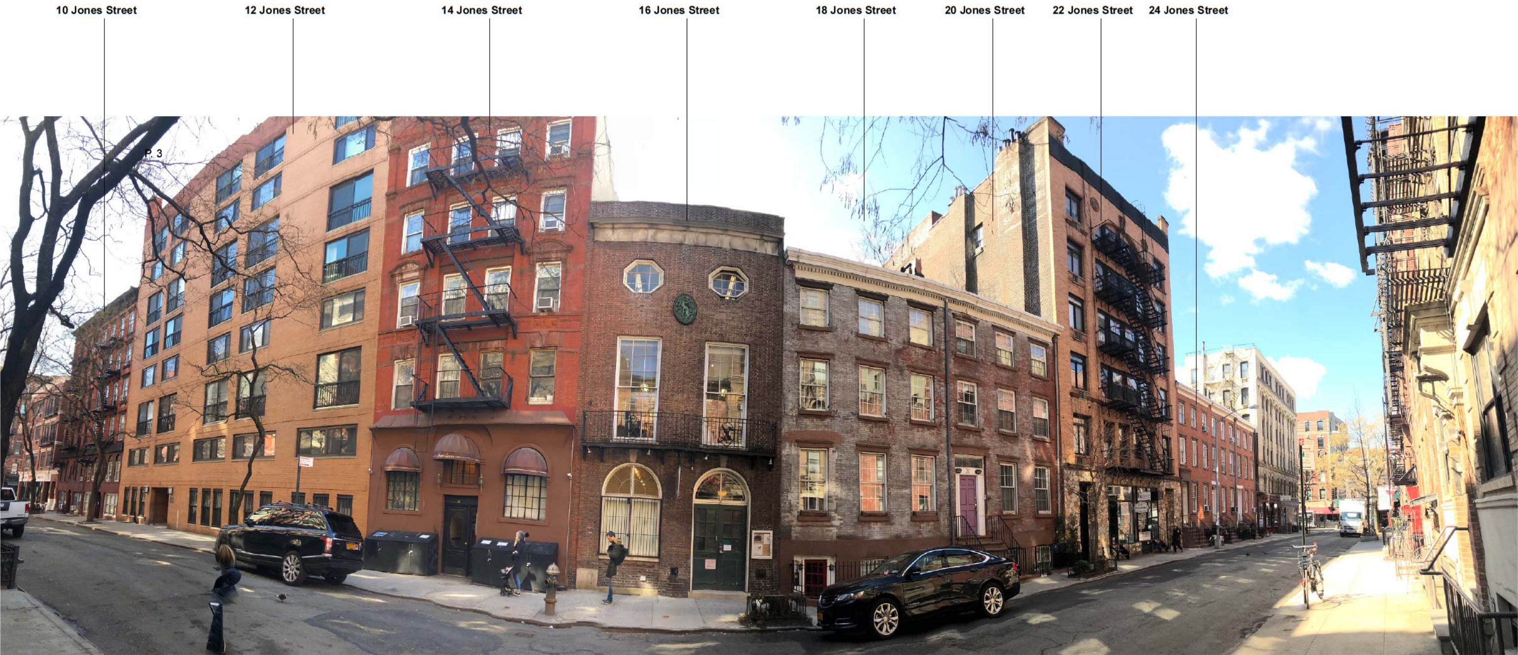
1. View of 16 Jones Street Facing South
